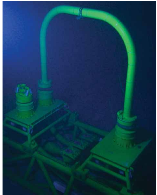
Completed HOOPS connection
