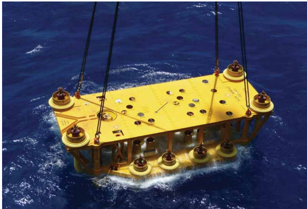
Installing a subsea manifold
