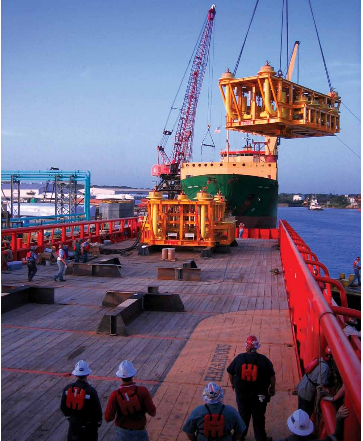
Load-out of the subsea manifolds
