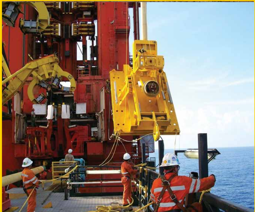
Pipeline End Termination (PLET) units like this one were installed at each end of the flowline.
