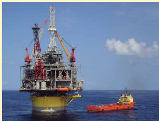
Helmerich & Payne's offshore Rig 205 rests tightly atop the Perdido Spar.
