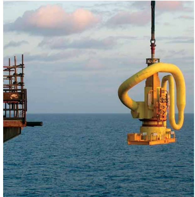
Installing an inlet assembly
