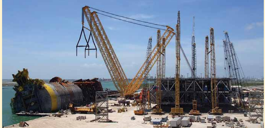
Perdido topside lift and spar hull at the KOS fabrication facility.
