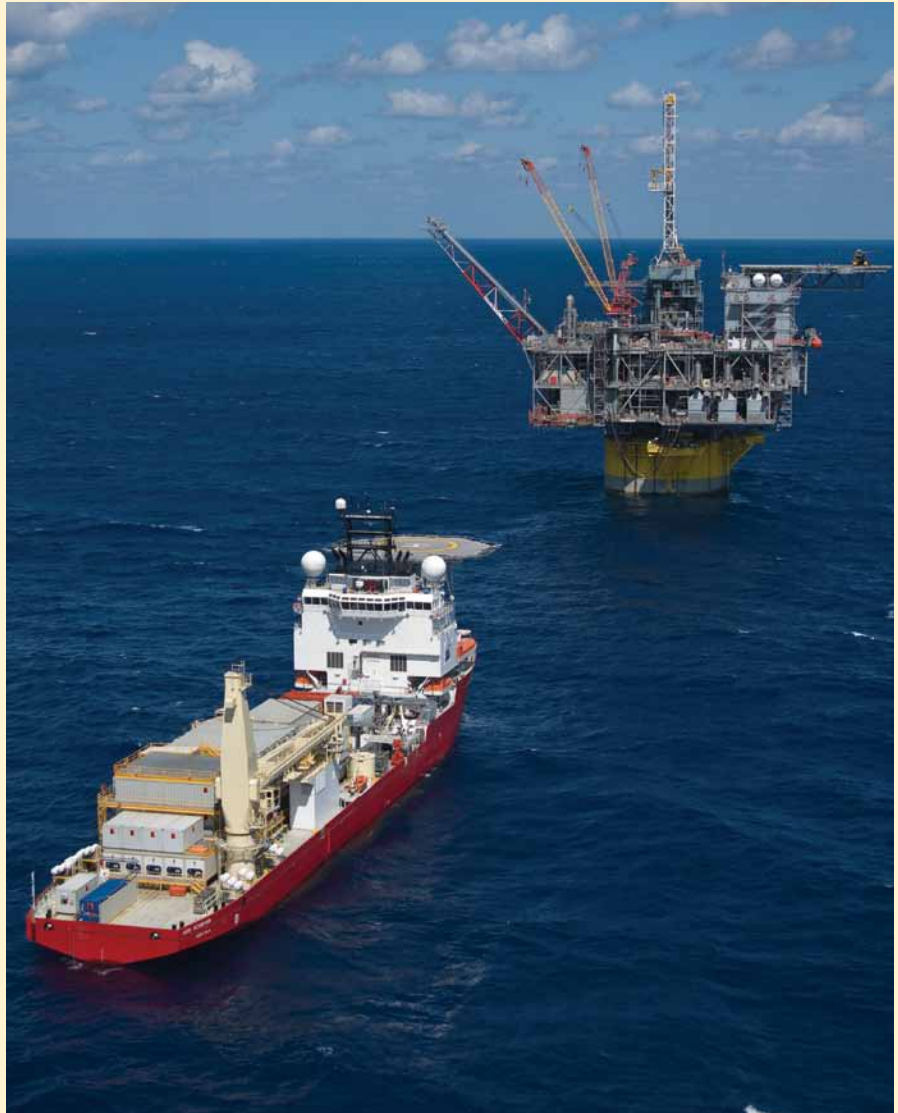
For more than eight months, the 430-foot DP-3 HOS Achiever MPSV served as Perdido’s floating hotel.
