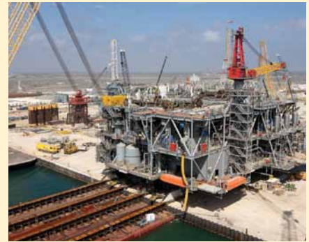
The Perdido topside loadout at KOS' facility.
