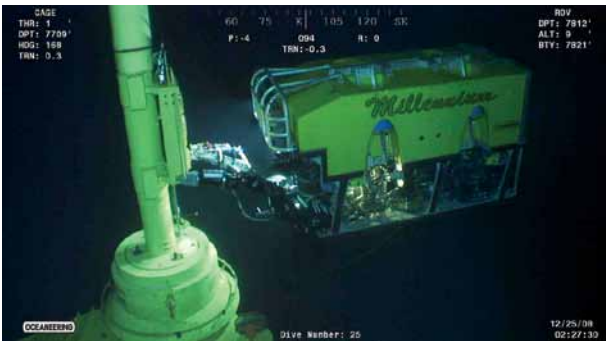
ROV-assisted installation of the flowline jumper
